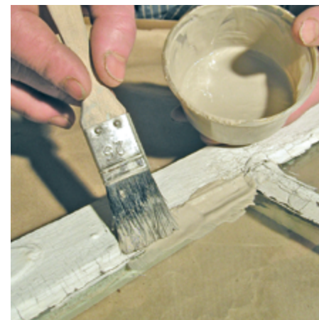
Thinned Putty temporarily seal cracked rebates.
