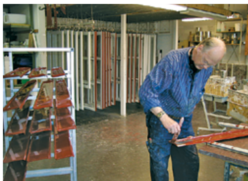
Painting windows and windowsills
