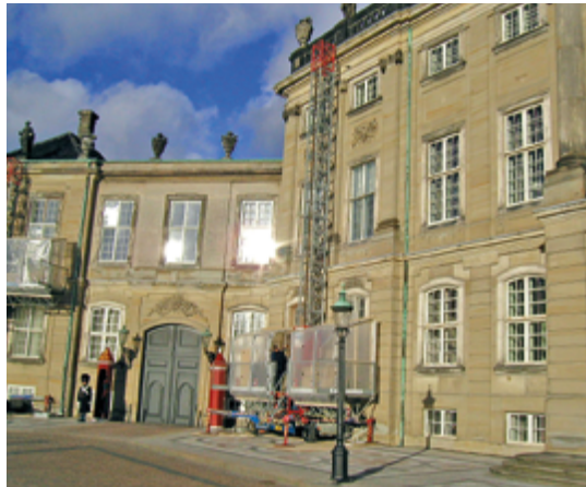
Allbäck Windowcraft and Paint for the Royal Castle, Copenhagen, Denmark.
