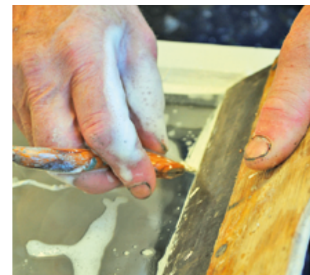
Wet the glass and cut in the paint
