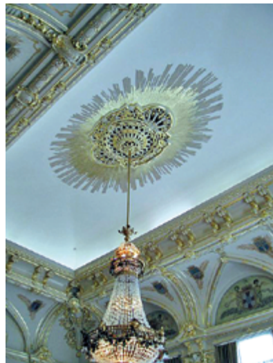
Masonic Lodge, Oslo, Norway. Linus Wallpaint on ceiling. Linseed Oil Paint on woodwork.
