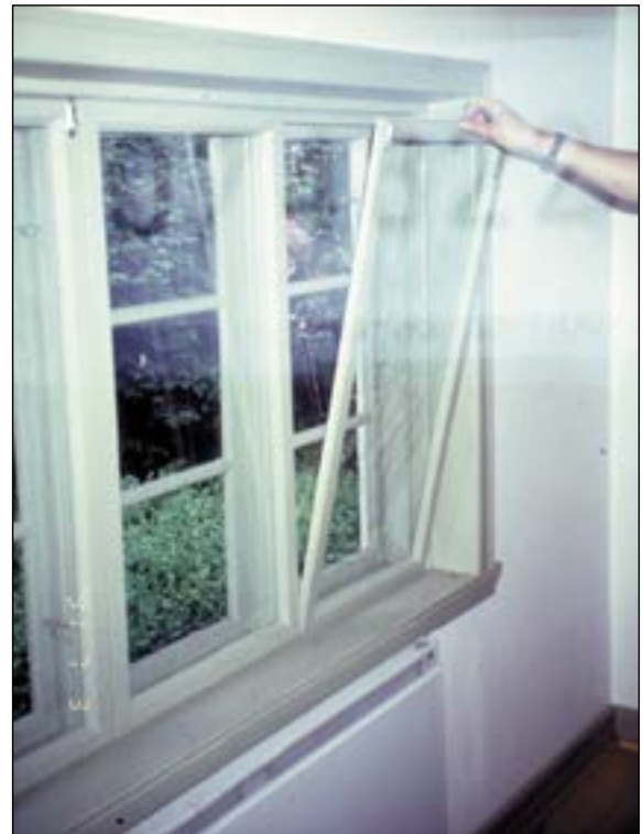
Linseed oil paint inside after 9 years First maintenance 2010
