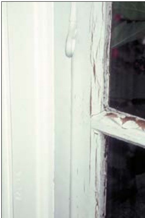
Alkyd paint inside after 2 years Repaired under guarantee
